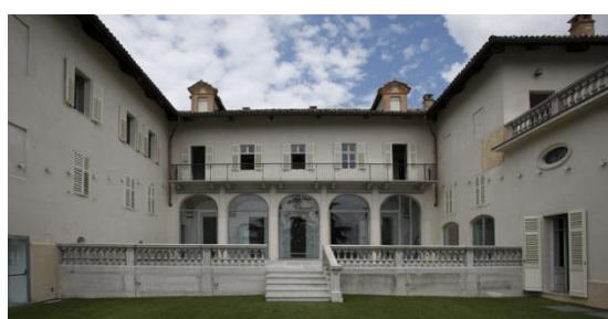
Palazzo Re Rebaudengo – Guarene (Cn)
